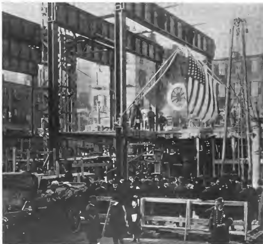
CEREMONIES OF LAYING THE CORNERSTONE OF THE A. C. A. CLUBHOUSE
